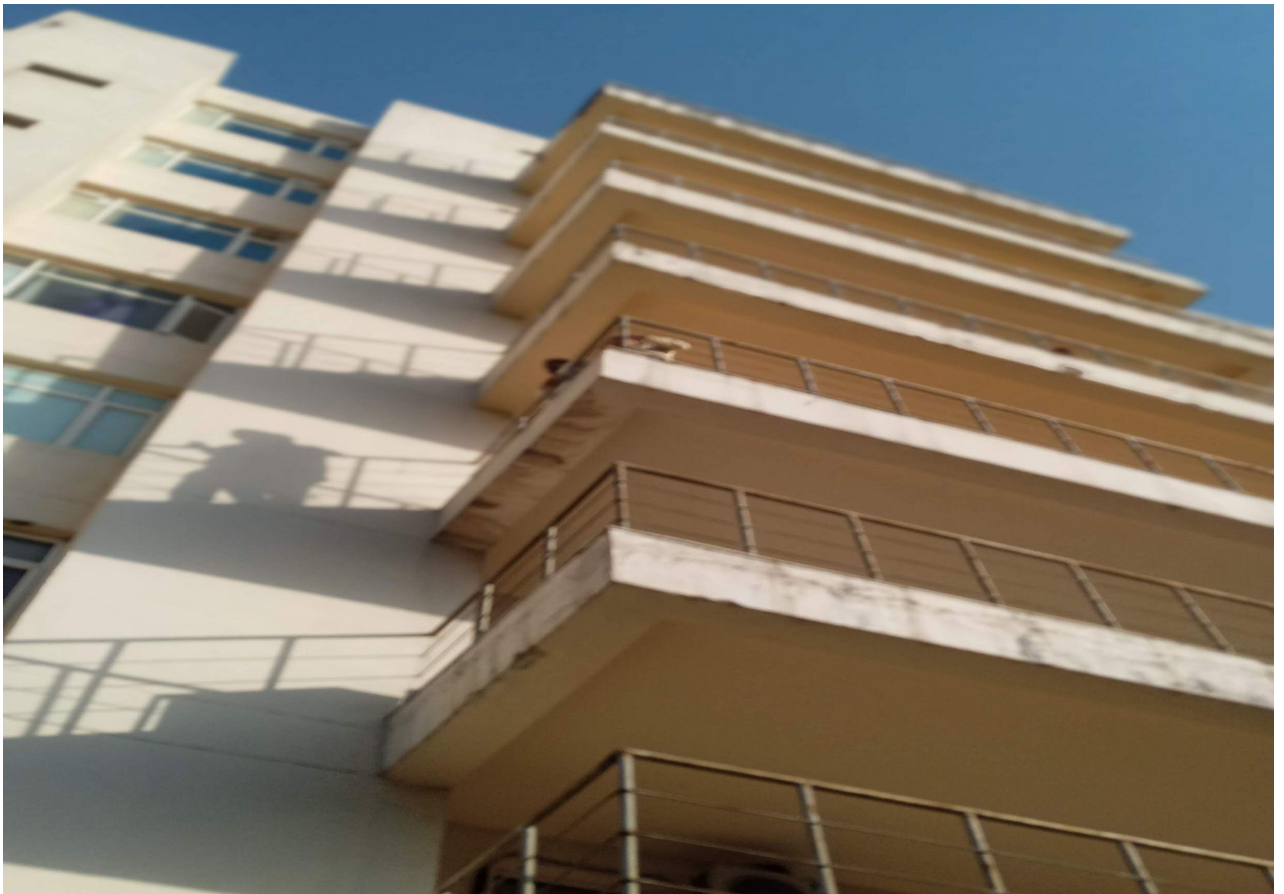
Photograph of Construction Building
